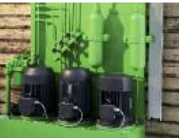
A high capacity hydraulic facility with accumulator ensures a proper shutdown when the mains fails or there is a disturbance.
